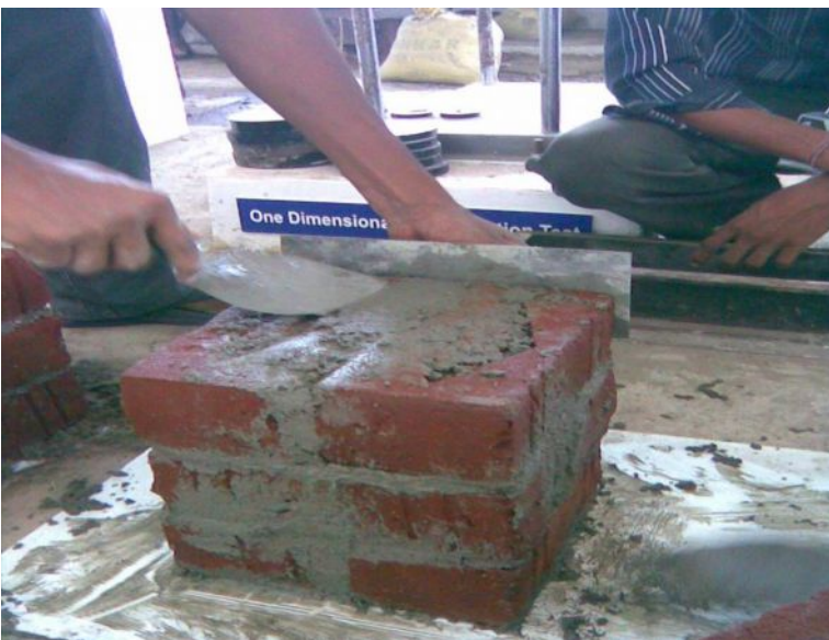
Fig 5 Photograph showing the construction of brick prism
