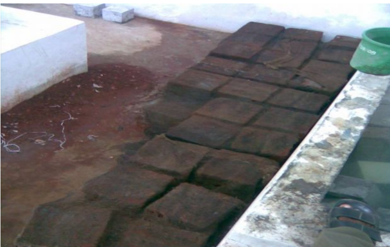
Fig 6 Photograph showing curing taken by using gunny bags
